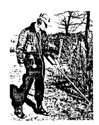
The GA-32 is unlike many other metal locators in that it detects the magnetic field of the marker. It will not respond to aluminum, brass, copper or other nonmagnetic materials. When the locator comes within range of an iron pipe or monument, a signal generated in the headphones guides the operator to the exact location. The GA-32 has a control so that its sensitivity can be adjusted over a very wide range to suit various situations.
